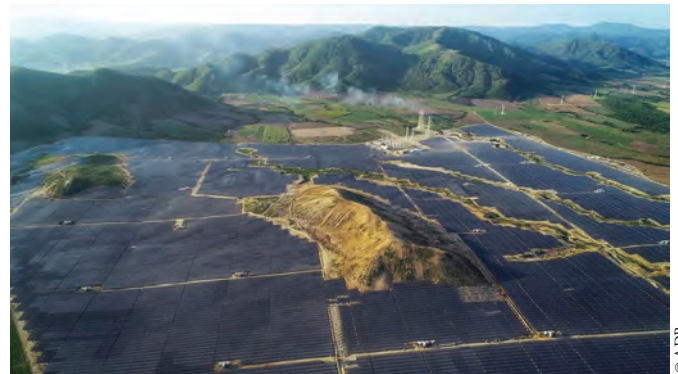
The new 257 MW facility is set to be the largest single operating solar power plant in Vietnam and one of the largest in Southeast Asia, helping to reduce 123,000 t of carbon dioxide annually.
