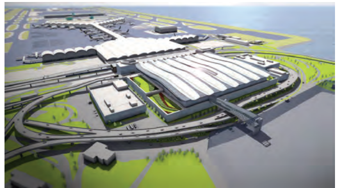
The expansion of HKIA Terminal 2 forms part of the airport's Three-runway System (3RS) project.
