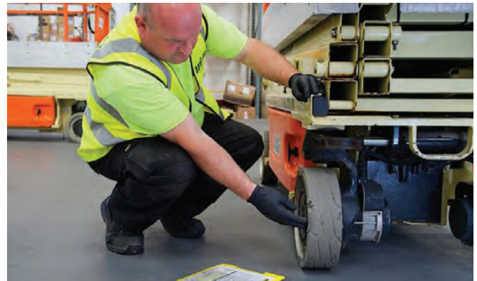
The virtual workshops will feature different equipment manufacturers each month, presenting the important points to consider when carrying out six or 12-month inspections on MEWP or MCWP equipment.
