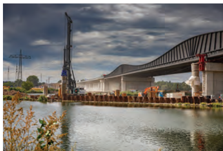
ABOVE AND LEFT: Liebherr LB 45 drilling rig at the rebuilding of the Neckartal Bridge. The machine has installed 106 foundation piles during the six-month piling work.
