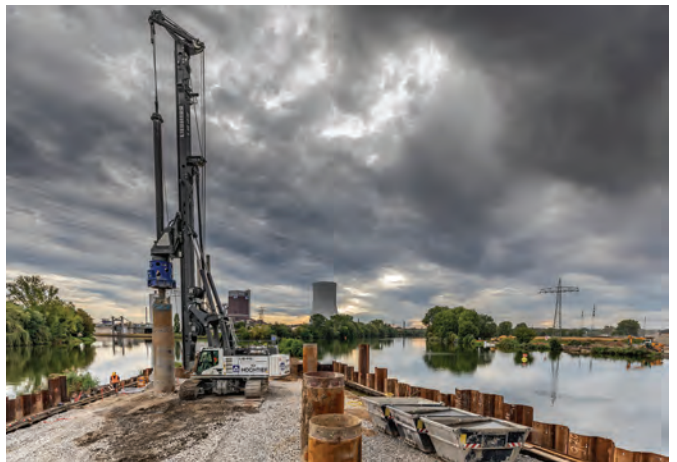
ABOVE AND LEFT: Liebherr LB 45 drilling rig at the rebuilding of the Neckartal Bridge. The machine has installed 106 foundation piles during the six-month piling work.
