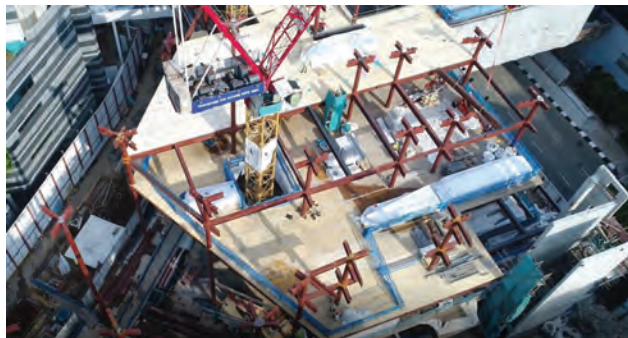
Single In-situ Column Splice
